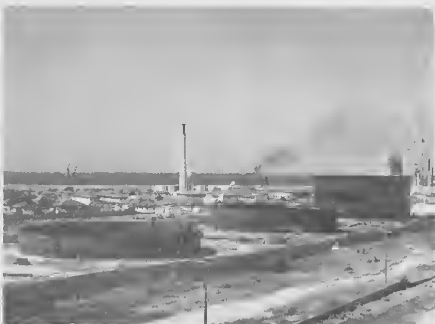
whole series of tanks that went up recently near the garage. Chicago Bridge, the contractors, chose to work on all six tanks simultaneously. ter un serie di tanki cu a worde erigi recientemente cerca di garage. Chicago Bridge, e contratistanan, a traha ariha tur seis tanki na mes
